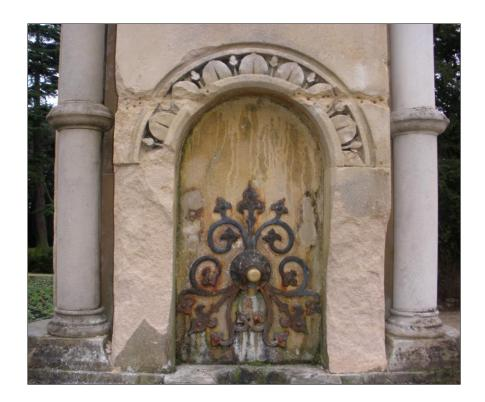
Spalling mainly affects the sides of the lower level block on the north face and the northern side of the lower level block on the west face where the upper level block now projects above it; there is cracking parallel to the stone surface on the north and west faces, showing where pieces will fall from in future. Spalling has also affected the upper level blocks on the north and west faces where they rest on the affected lower level blocks.
