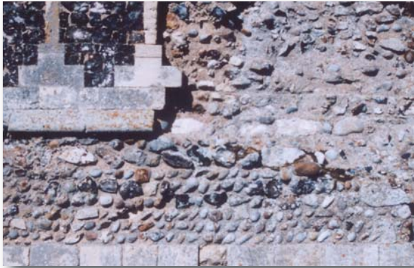
The flint rubble wall at Leiston Abbey.
