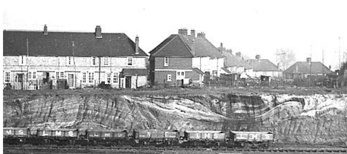
The railway cutting at Hadleigh Road - widened in May 1933.
